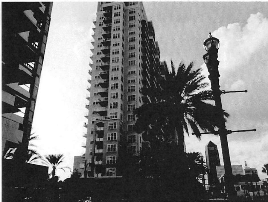
Adjacent condo tower to the west
