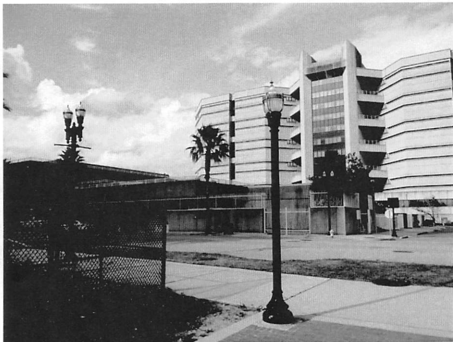
Jacksonville Sherriff Office building to the north
